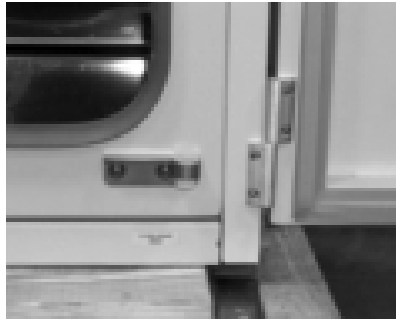
Figure 6-19. Bottom Inner Door Hinge
